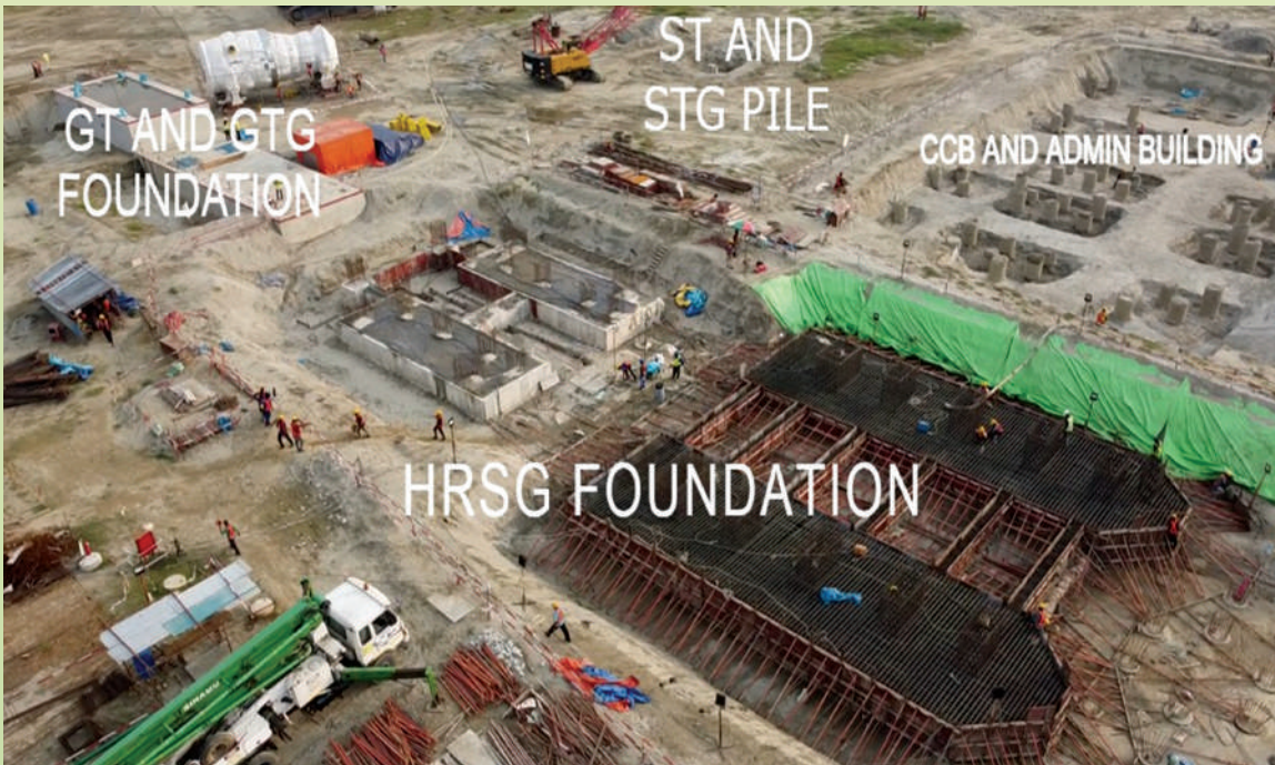
Major Construction at Site
