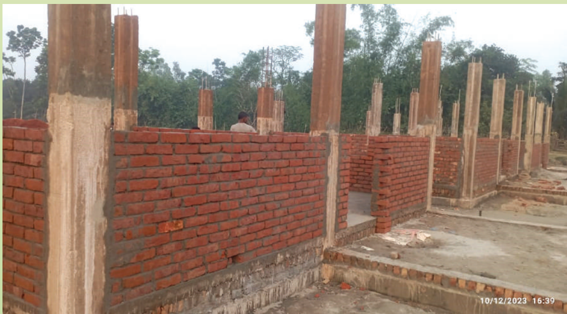
Construction of resettlement houses in the Resettlement Area
