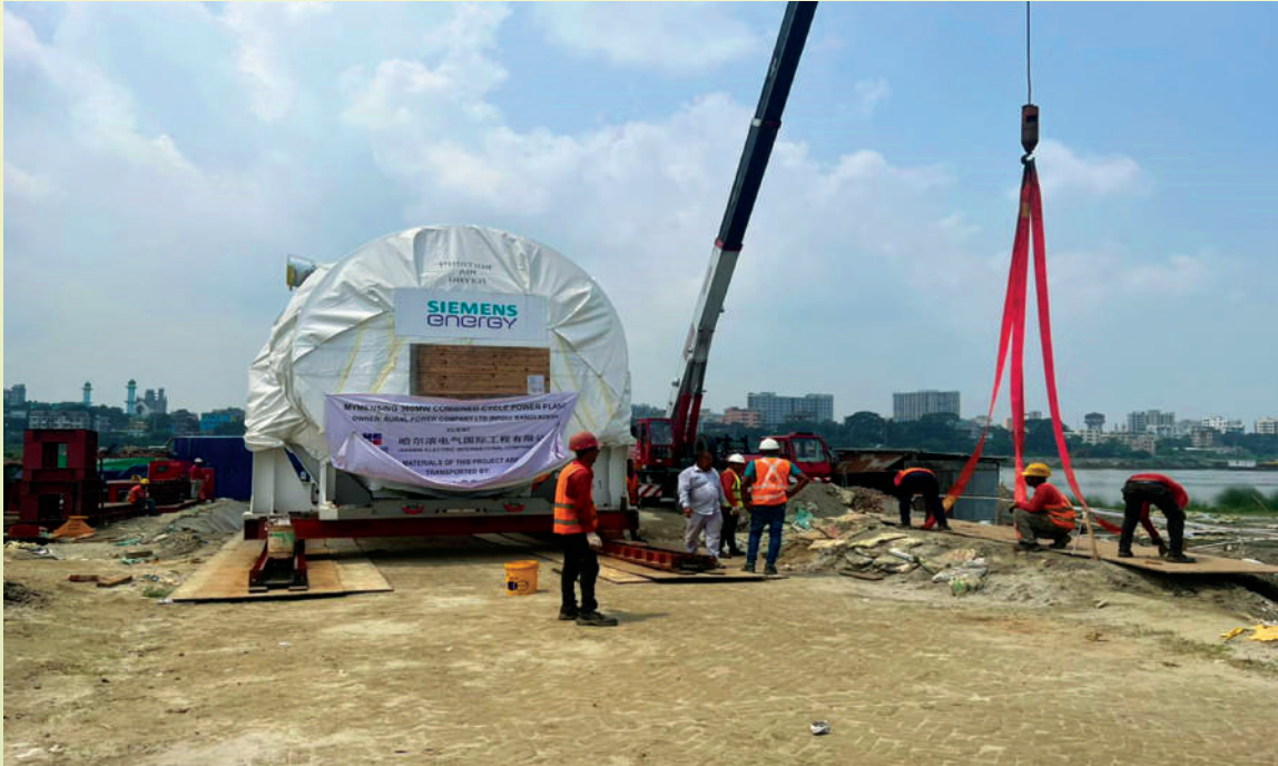
GT unloaded at site
