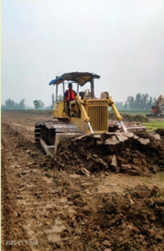
Land Development works of the project
