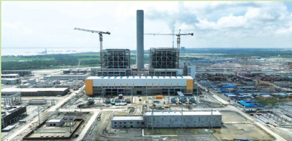
Boiler Turbine Generator area [Superstructure works]
