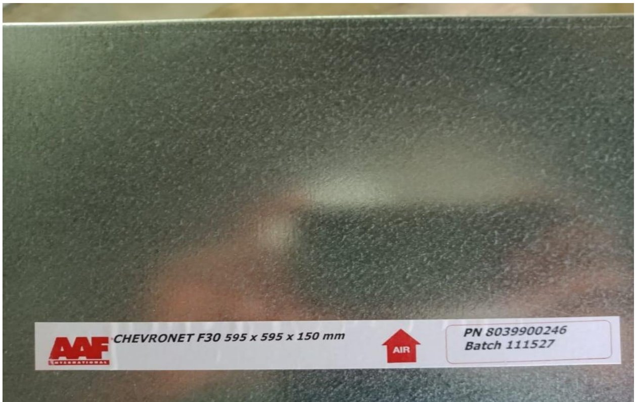
Picture 3 & 4: Charge Air filter nameplate of Raozan Power Plant.
