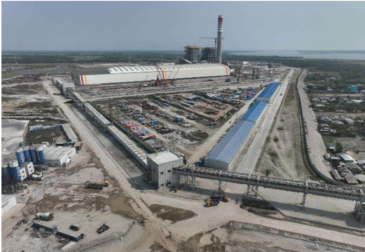
Coal Conveyer Belt and Transfer Tower (Structure Works)
