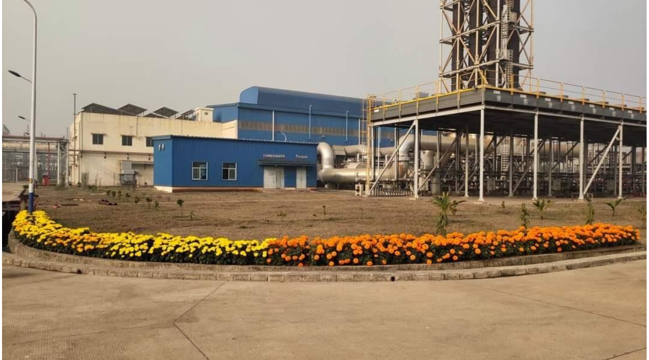
GAZIPUR 105 MW HFO FIRED POWER PLANT
