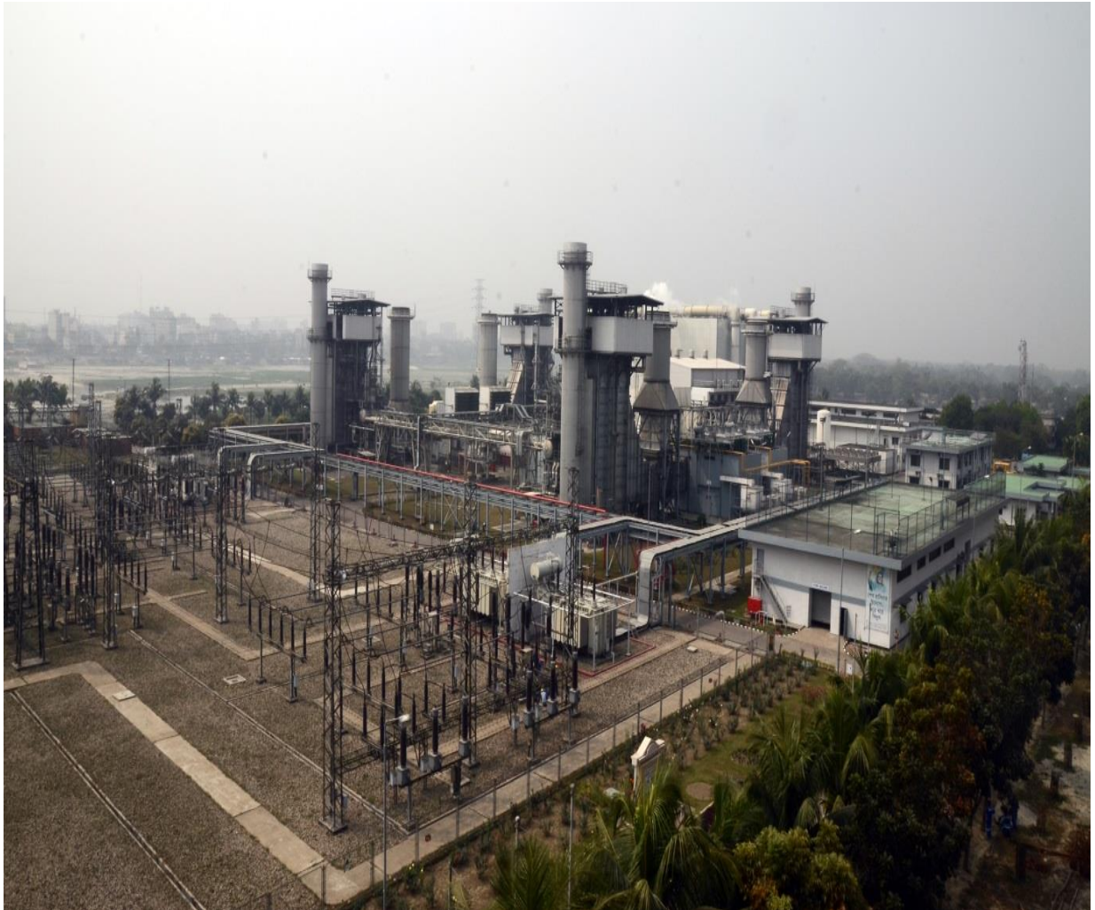
MYMENSINGH 210 MW COMBINED CYCLE POWER STATION
