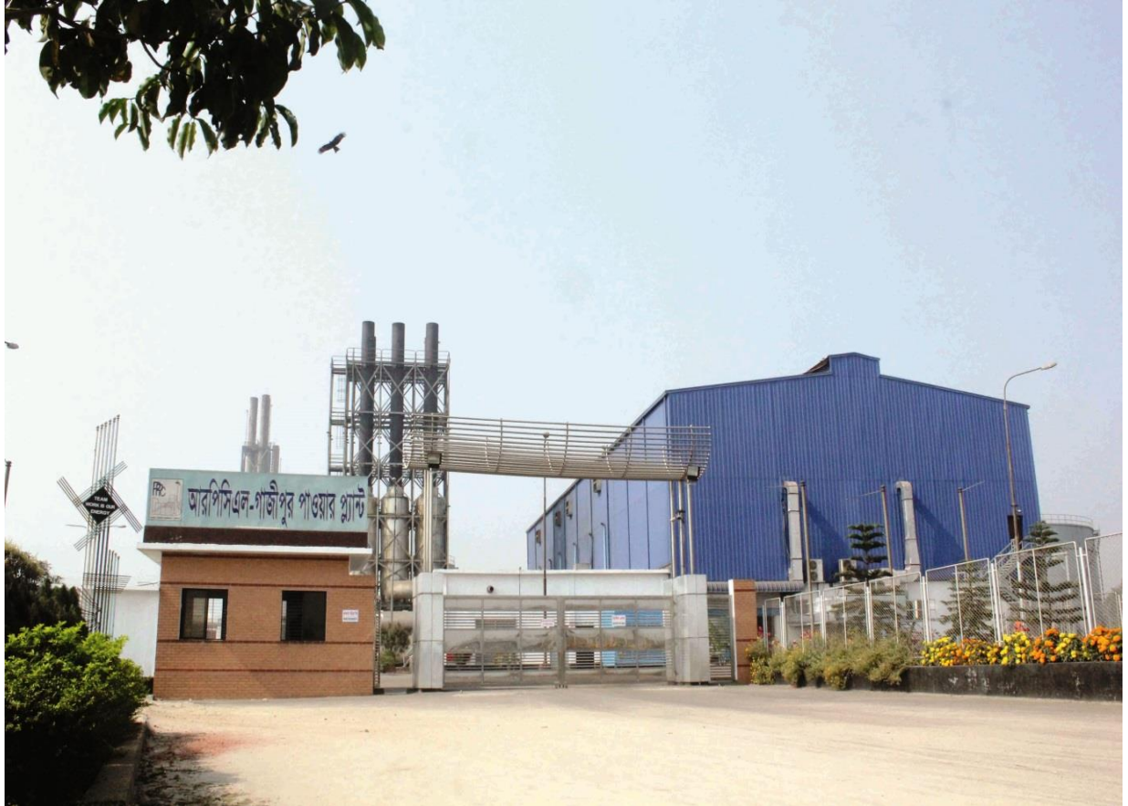
GAZIPUR 52 MW DUAL-FUEL POWER PLANT
