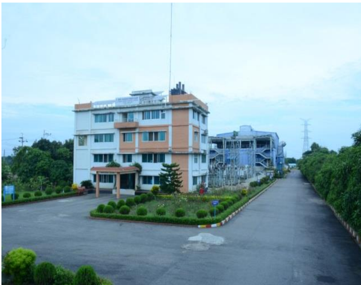
RAOZAN 25 MW DUAL-FUEL POWER PLANT
