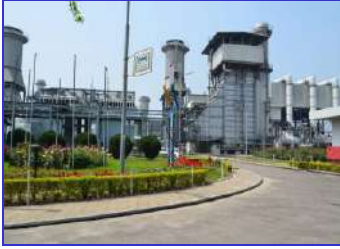
Mymensingh 210MW Combined Cycle Power Station
