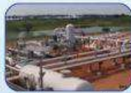
Bhola gas pipeline
