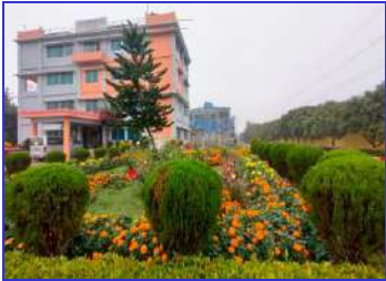
Raozan 25 MW Dual-Fuel Power Plant
