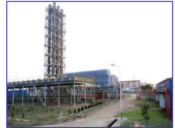
Gazipur 105 MW HFO Fired Power Plant
