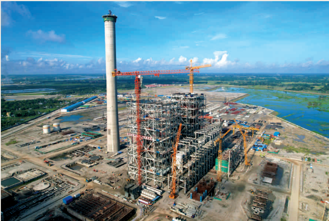
Overview of Patuakhali 1320 (2x660) MW Coal Fired Thermal Power Plant Project
