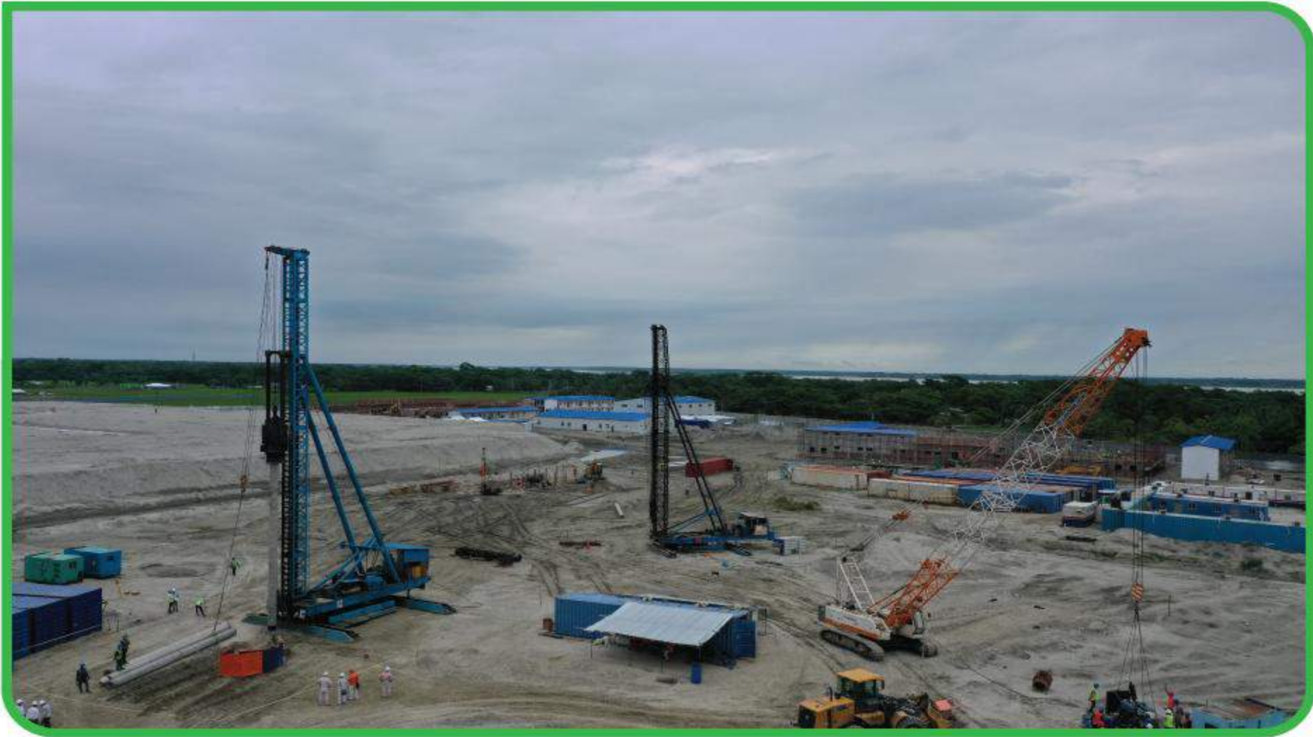
Piling Storage and Construction Works of Patuakhali 1320 (2x660) MW Coal Fired Thermal Power Plant Project, Kalapara, Patuakhali.
