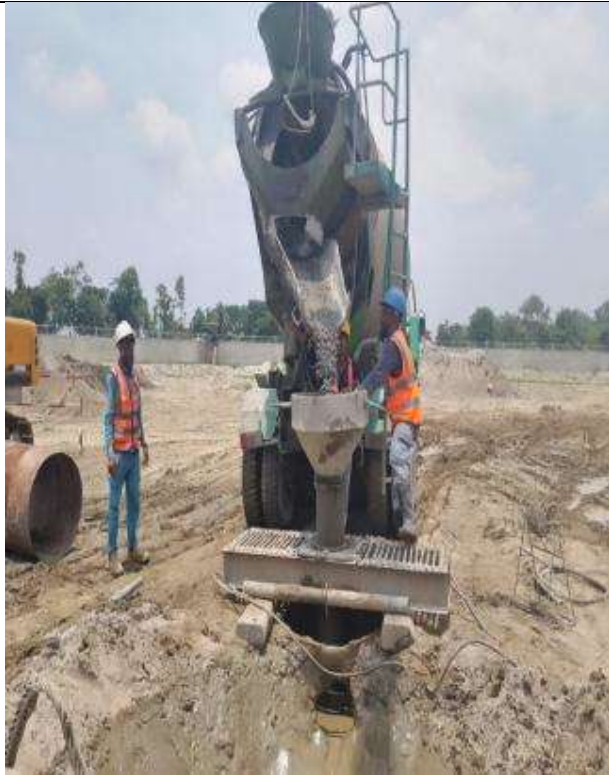
Casting of Pile of Different Structure.
