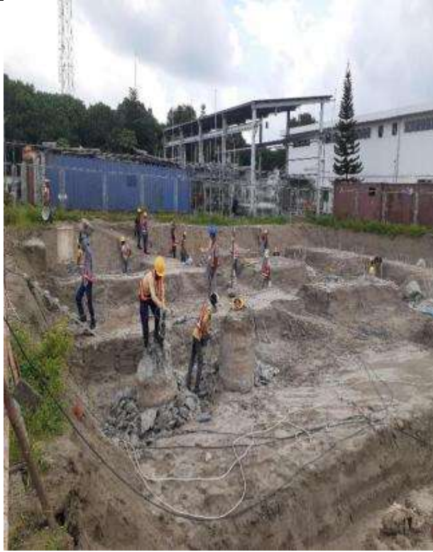
Workshop & warehouse building foundation pile cap exposure ongoing
