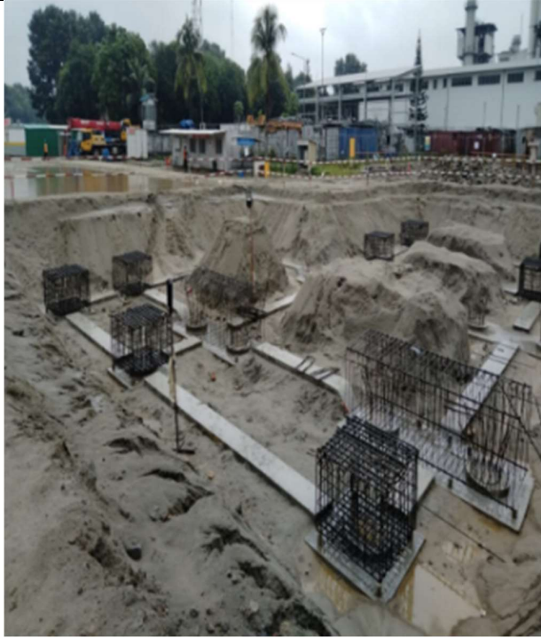
UNIT Switchgear Building foundation rebar work ongoing
