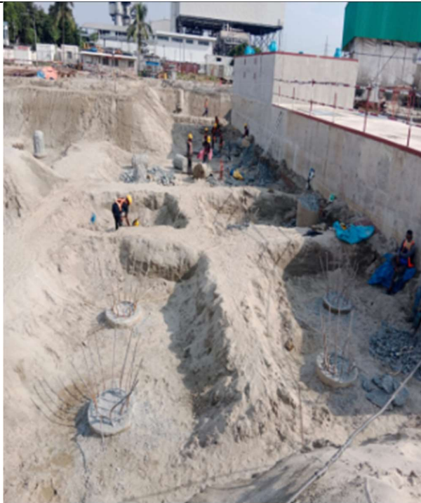
GT Hall Earth Excavation for Pile-head exposure and breaking ongoing
